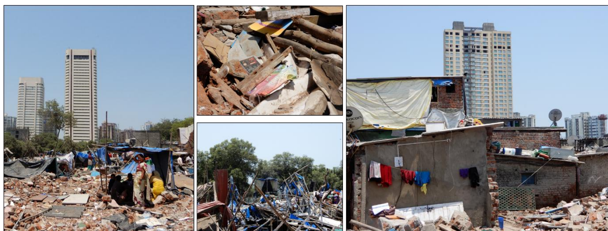
Rubble at Ambedkar Nagar post demolitions seen in the backdrop of Cuffe Parade's famous World Trade Centre (L); A child's school textbook lying amidst the rubble (top-C); Remains of people's homes amongst the mangroves (bottom-C); The infamous Adarsh Housing Society building as seen from the demolition site, which still stands tall in spite of its illegality (R)
