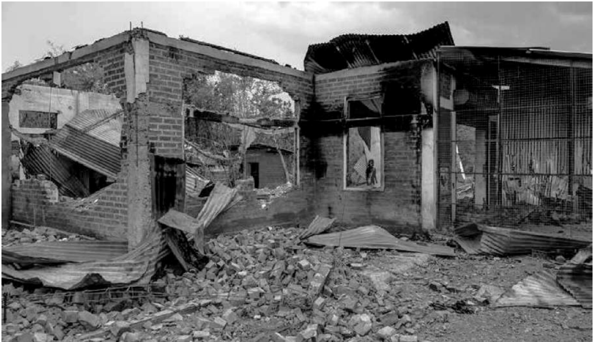
Burnt down houses in churachandpur district, on 31 May
