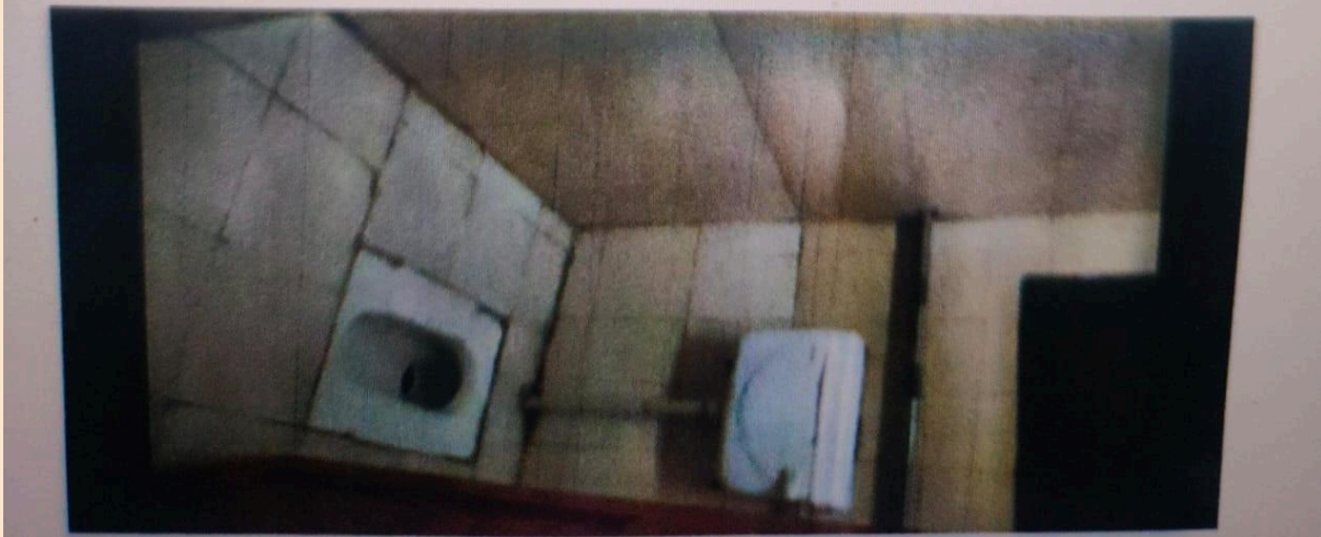
Photo of the repaired toilets that were shared by the DUSIB
